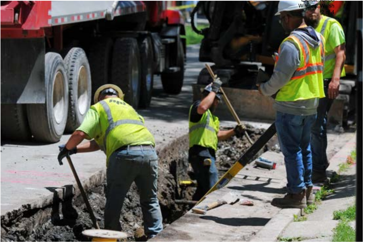
Peoples Gas workers installing a new natural gas pipe in Albany Park in 2019. The utility is replacing deteriorating gas pipes under a program that's scheduled to take until 2040 to complete. | VICTOR HILITSKI / SUN-TIMES FILE
